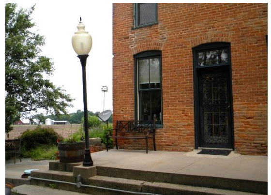
Figure 3: Former general store in River Junction. Photo Credit: Johnson County PDS, 2019.
