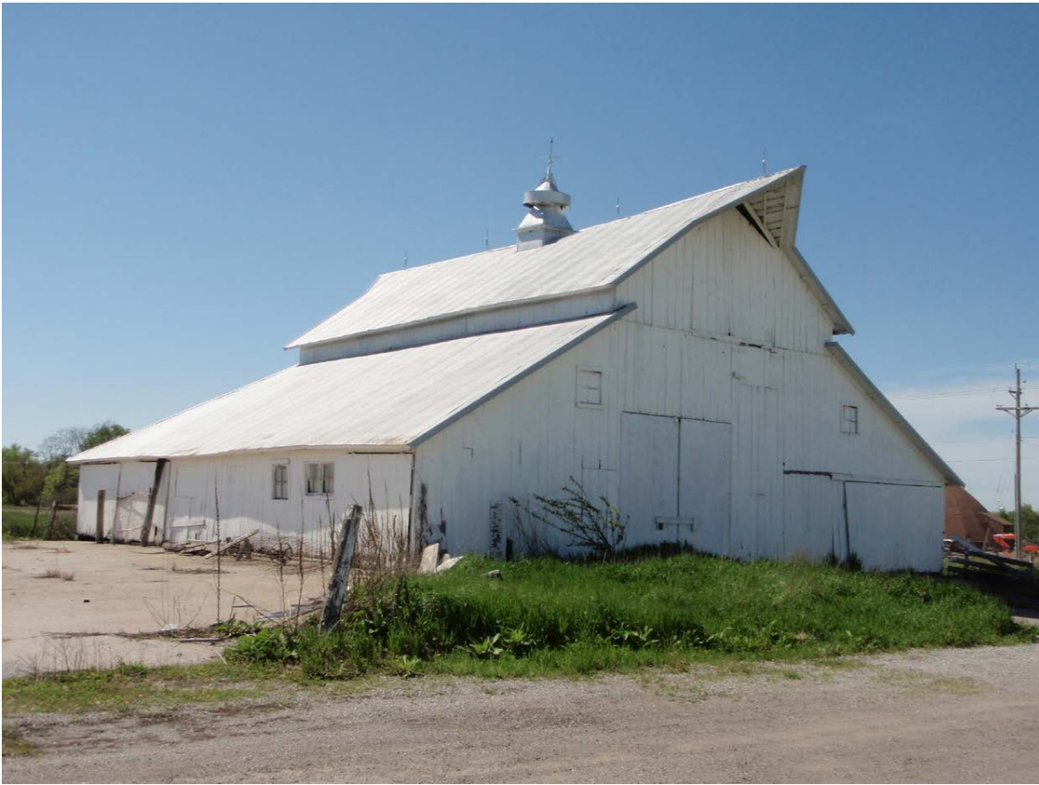
Monitor-roofed stock barn exterior
