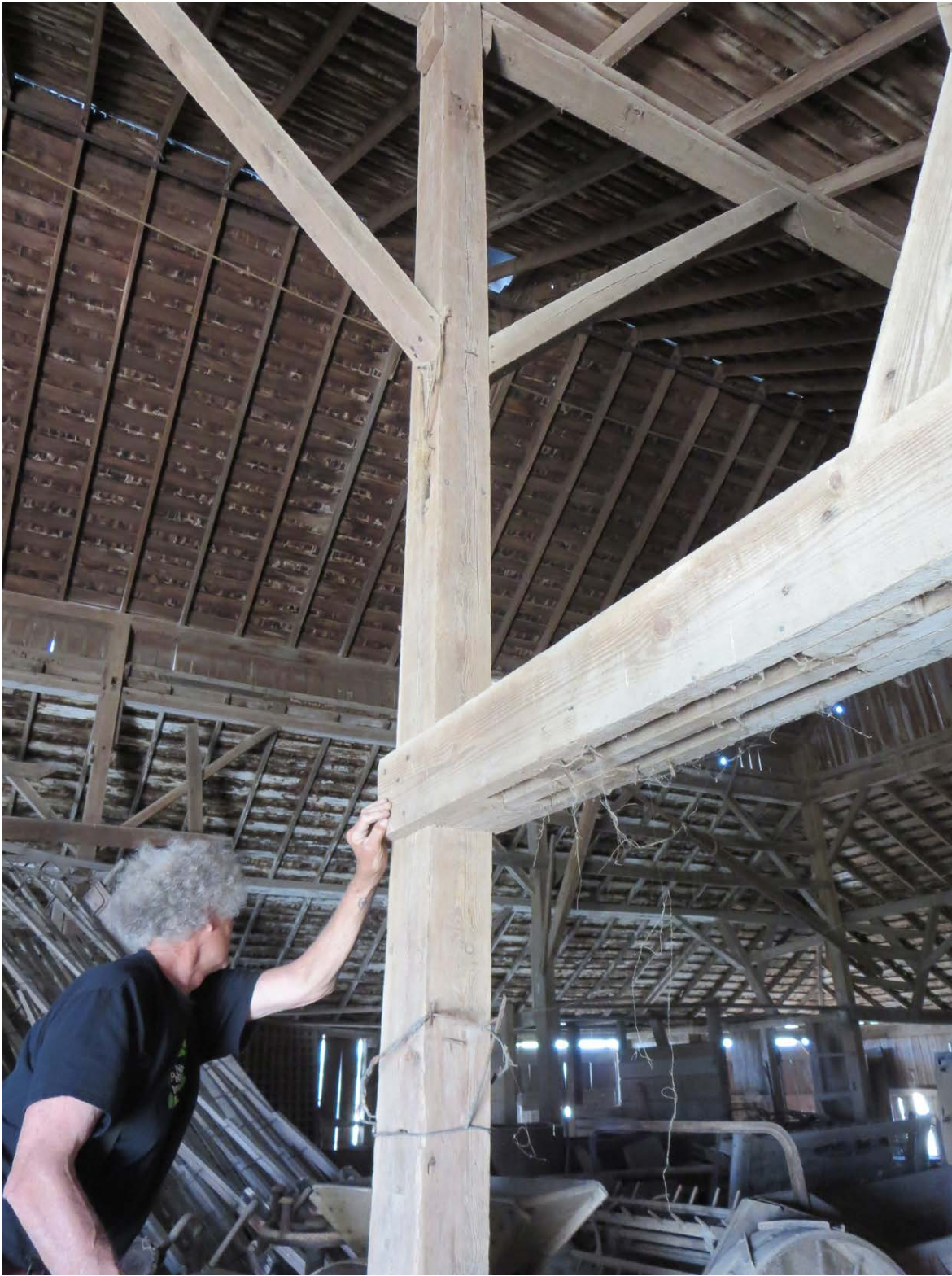
Investigating missing beams, view of roof interior
