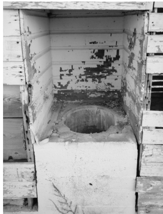
Metal basin built into east side of Crib
