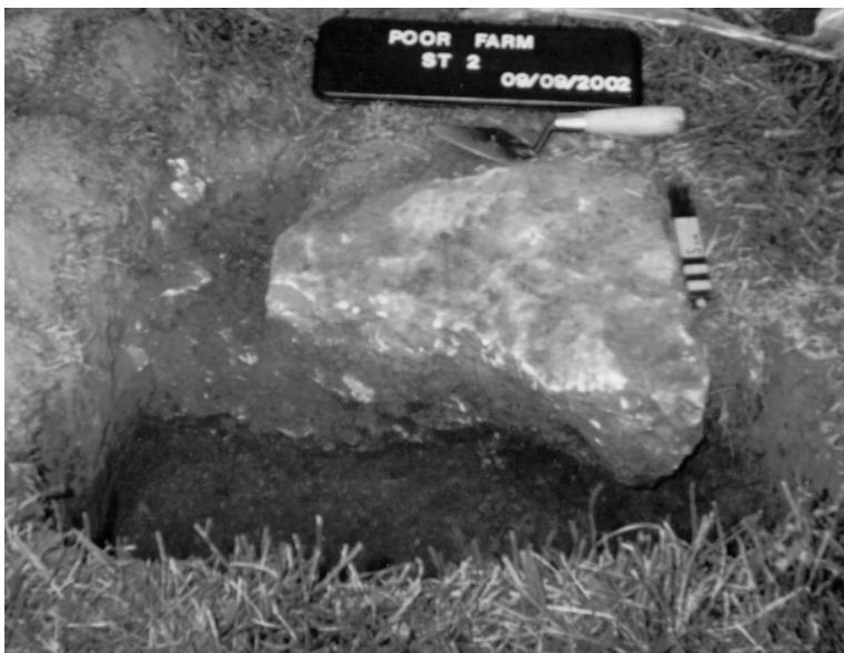
Figure 13. Photograph of intact limestone foundation wall uncovered in 2002 just north of the NW corner of the extant asylum building, Site 13JH1148 (Rogers 2004). Left photo: view is to the East; Right photo: view is to the North.
