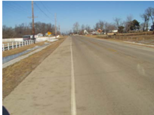
Paved shoulder, Sand Road
